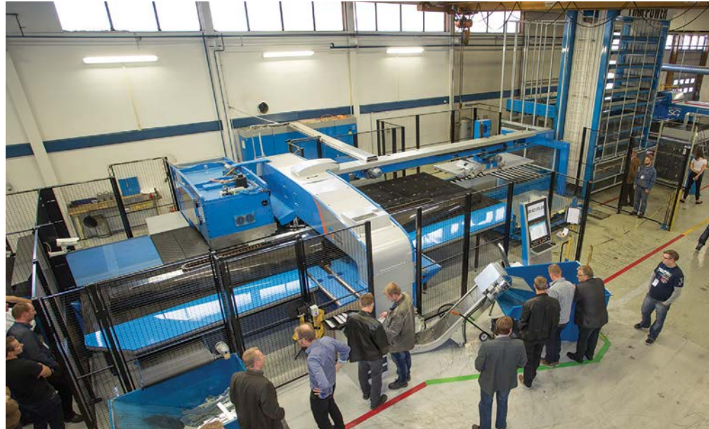
The new machine was installed in the existing automatic sheet warehouse, and overall, the project succeeded better than anticipated. Thirty-hour production runs on the SBe began immediately.
