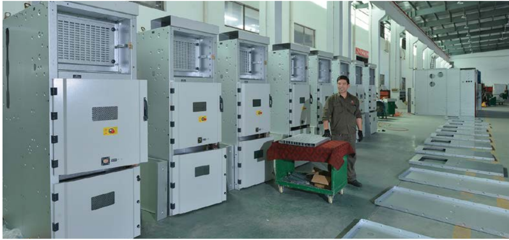
Tian Xiang is one of the most successful Chinese companies currently operating in the electrical cabinet industry.
