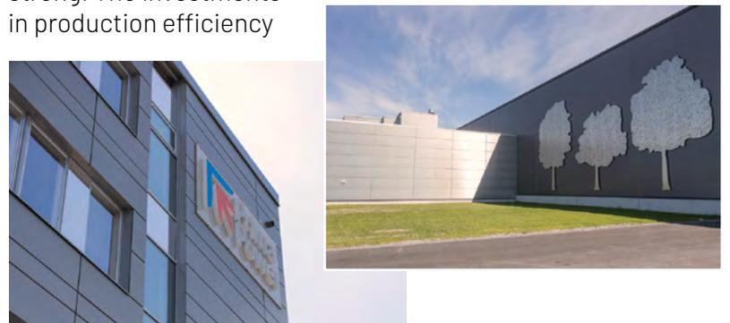
The façade panels of the new Prima Power Seinäjoki factory were manufactured by PRP on Prima Power machines.
